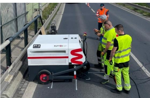
Repair using the “microwave patcher” FT-3
