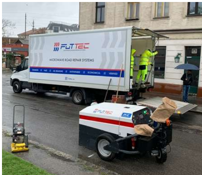
Repairs of potholes with FUTTEC® microwave technology in Vienna
